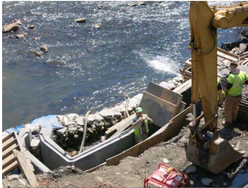
Construction begins at 182nd Street dam! (NYCDPR).
