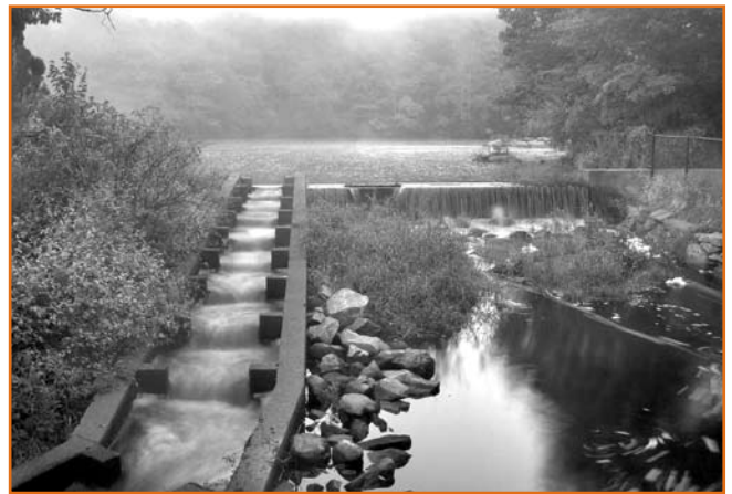
Computer rendering of an operational fish ladder on the left. Reservoir with dam is in the background. Image courtesy of Alexey Sergeev
