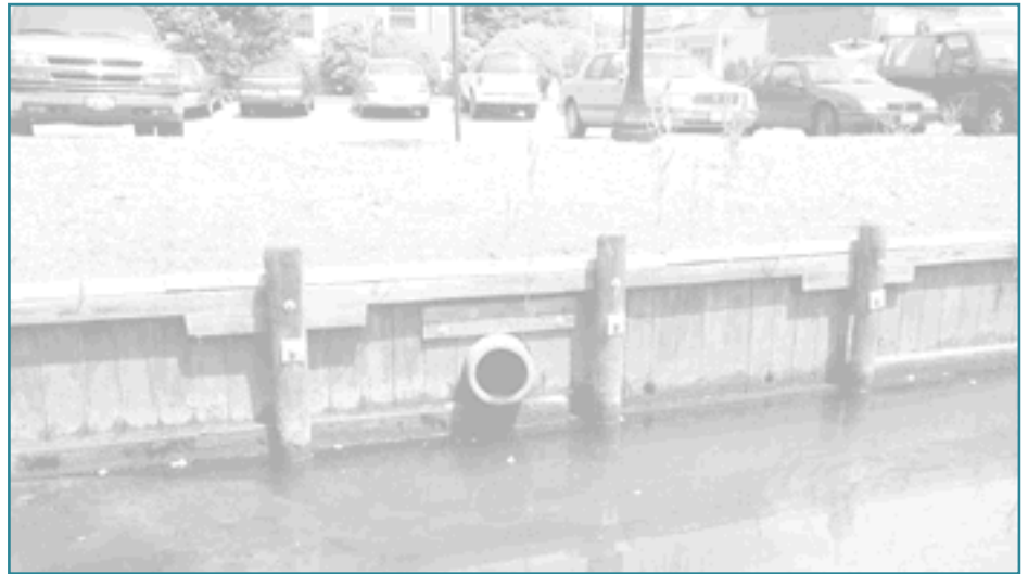
After stormwater enters a municipal separate storm sewer system it is released into a local waterbody. Photo courtesy of New York Sea Grant, Eileen Keenan
