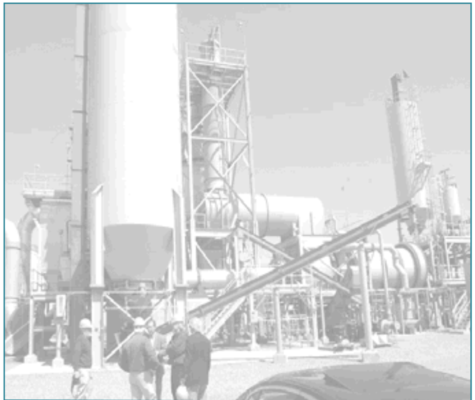
Gas Technology Institute - thermo-chemical rotary kiln facility.
